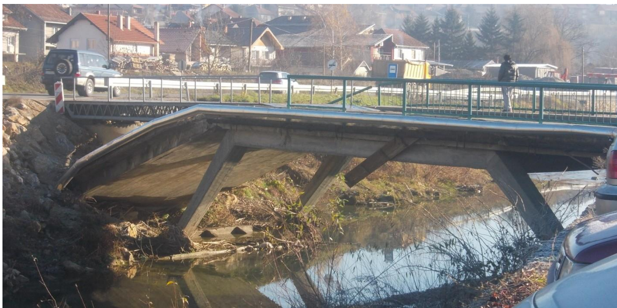
Picture 03: Bridge 02, demolished by the floods and temporary adapted
