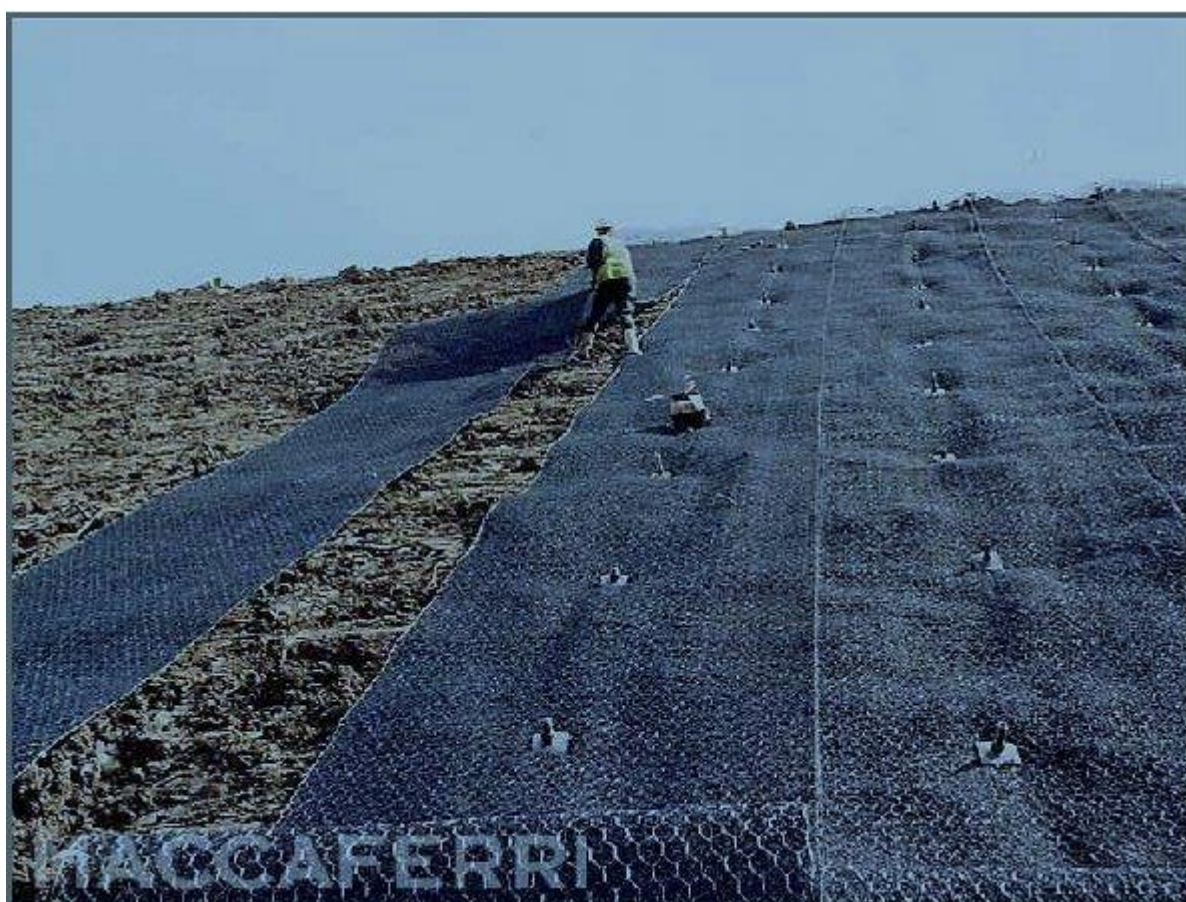
Figure 2 - Similar construction works with geocomposite covering a river bank
