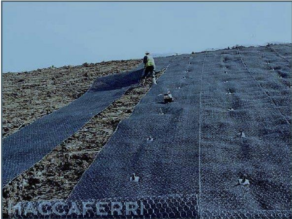
Figure 2 - Similar construction works with geocomposite covering a river bank
